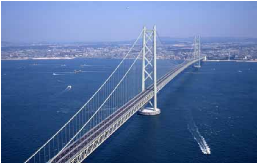
[Akashi-kaikyo Bridge] completed 1998 Type : 3-span continuous 2-hinges stiffening truss suspension bridge Bridge length : 3,911m (960m+1,990m+961m)
