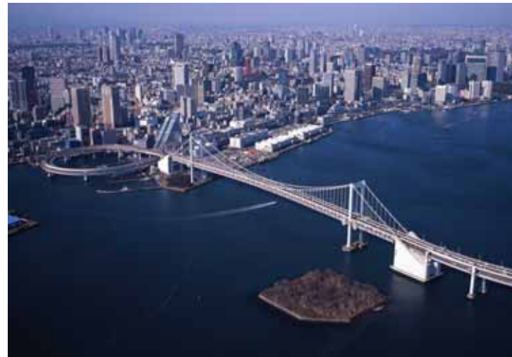
[Rainbow Bridge] completed 1993 Type : 3-span continuous 2-hinges stiffening truss suspension bridge Bridge length : 798m (111.5m+570m+111.5m)
