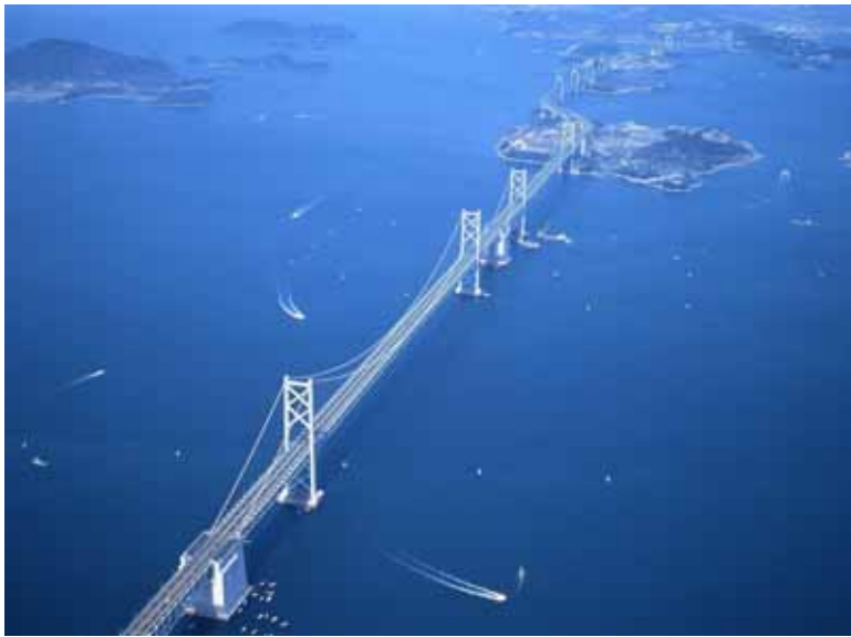
[Minami Bisan-seto Bridge] completed 1988 Type : Suspension bridge, double deck (Highway and railway) Bridge length : 1,628m
