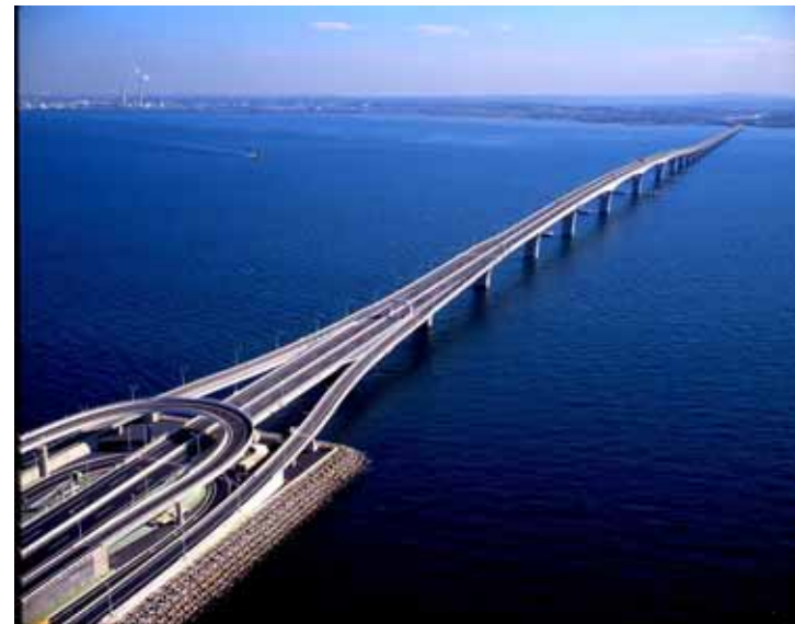
[Tokyo Bay Aqua-Line Bridge] completed 1995 Type : Continuous steel box girder bridge Bridge length : 4,384m
