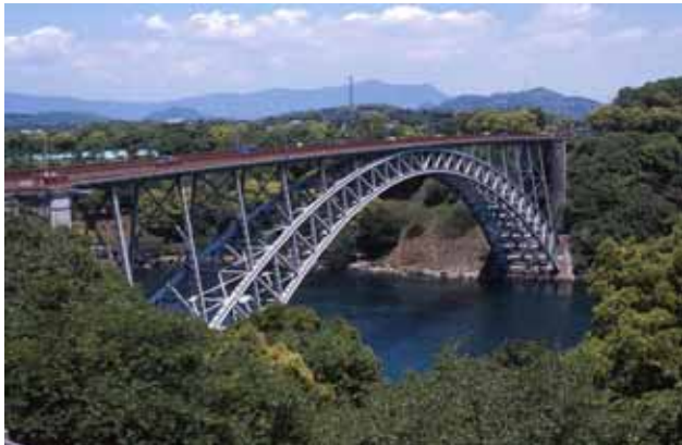
[Saikai Bridge] completed 1955 Type : Fixed braced arch Bridge length : 244m
