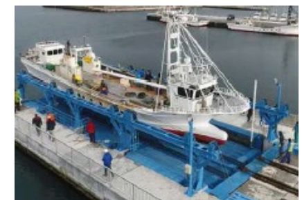
Ship-lifting equipment at Oarai Fishing Port
