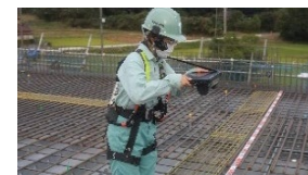
Bar arrangement inspection using AI
