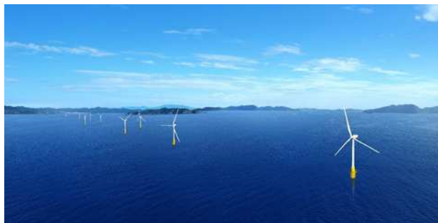
Japan's first floating offshore wind Turbine facility put to practical use in Goto City, Nagasaki Prefecture (Referenced from Toda Corporation official website)
