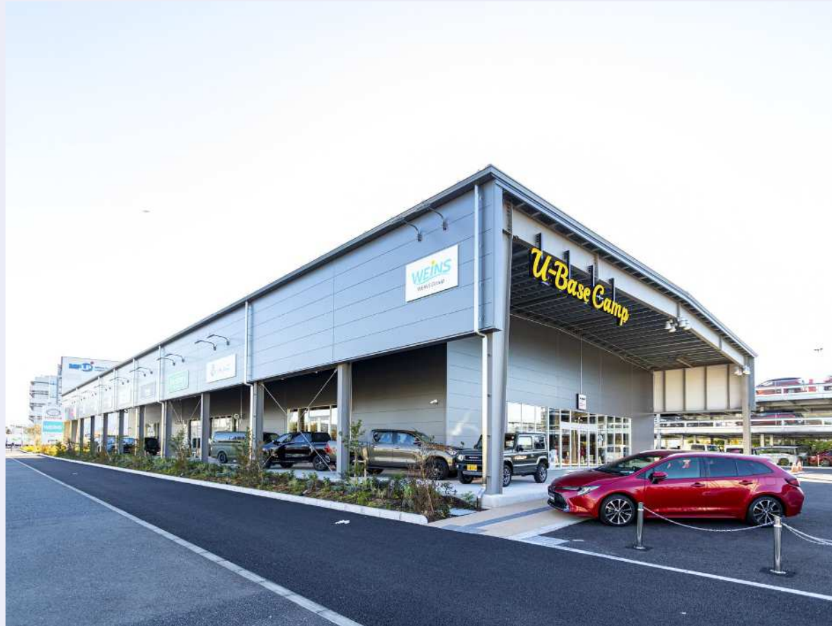
WEINS PARK Ebina U-BASE building
