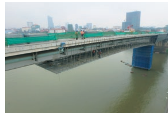
Installation of panel scaffolding for repair and painting of Chroy Changwar Bridge
