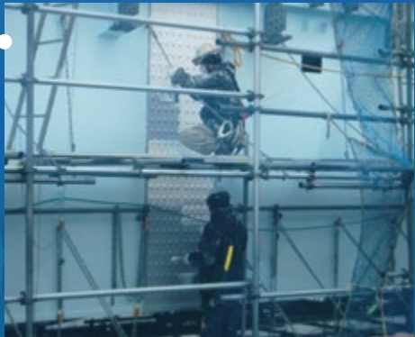
The joints between the blocks are painted on-site the same as in the plant.
