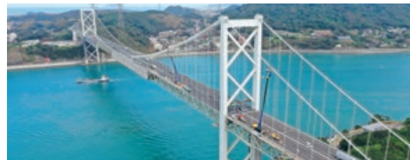
Installation of work scaffolding on a main cable using a vehicle for work at height
