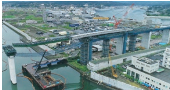
Incremental launching construction (The part that is temporary support diagonally upward at the end of the girder on the left side of the photo is the "curvature handling device.")
