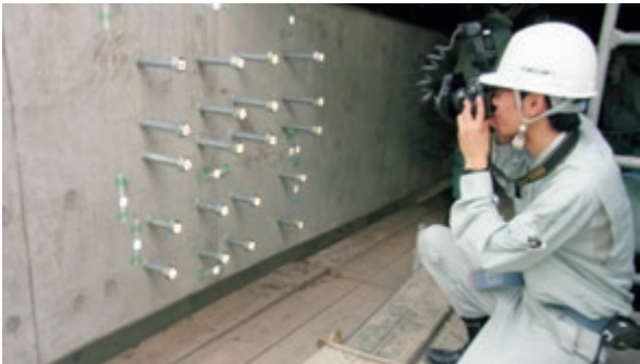
“Anchor version VFORM,” an example of 3D measurement of anchor bolt position
