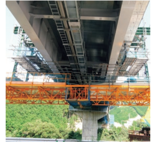
Mobile scaffold for scaffolding disassembly
