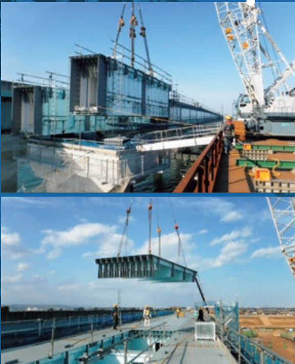
One by one, the assembled blocks are lifted into place using cranes, etc., and assembled into a bridge.
