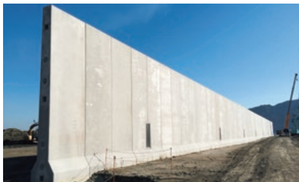
Steel-concrete composite precast seawall
