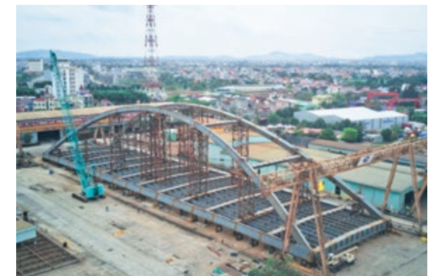
Temporary assembly of Kalna Bridge at in Vietnam production plant
