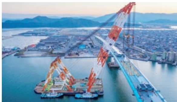
Large block erection using a crane vessel
