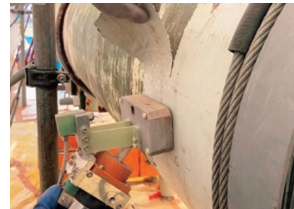
Expanding the application of a paint removal method (application to a main cable of the Kanmon Bridge)
