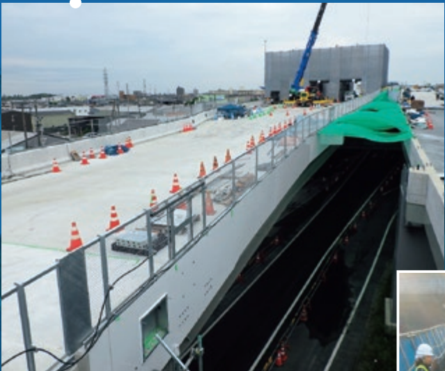
A deck that vehicles can travel on is built on top of the erected steel girders. The material is mainly reinforced concrete, but there are also steel decks manufactured from steel plate in plants.
