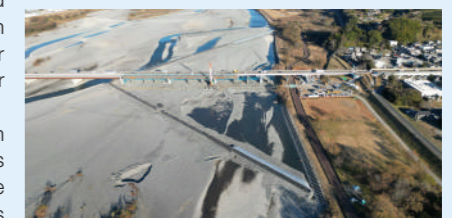
Erecting bridge girders in the river
