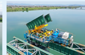
Launching nose rotating equipment
