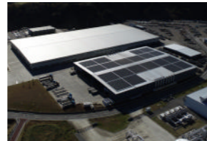
A solar power system installed at the Yokogawa System Buildings' Mobara Plant
