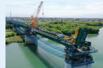
Rotating the launching nose
