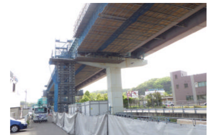
Okishin Viaduct, Sasebo Road
