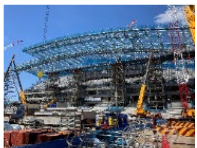
Construction of a football stadium in Hiroshima
