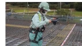
Bar arrangement inspection using AI
