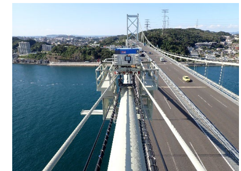
Photo provided by: West Nippon Expressway Company Limited
