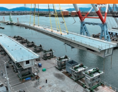
Connection with column members on the quay
