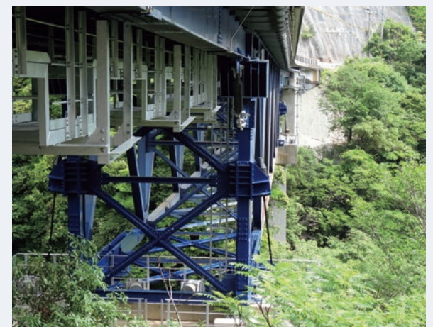
Buckling restraining braces installed on the Senjin Bridge
