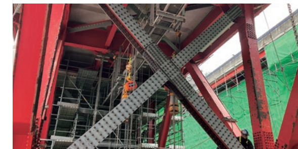
Anogawa Bridge anti-leaning structure reinforcement
