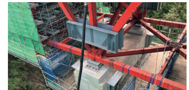
Anogawa Bridge bearing replacement completed
