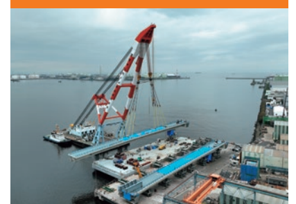
Launching work (loading onto barge)
