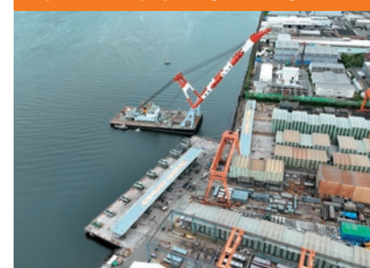
Lateral transport from the ground assembly yard to the quay using a floating crane
