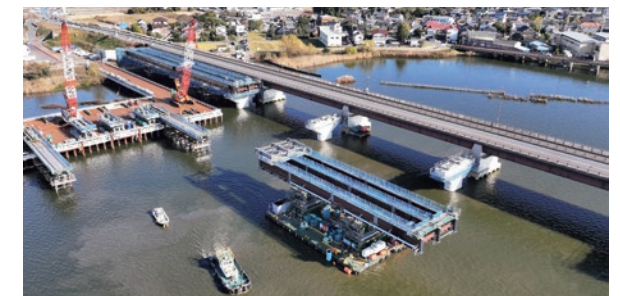
Jingubashi Bridge barge erection
