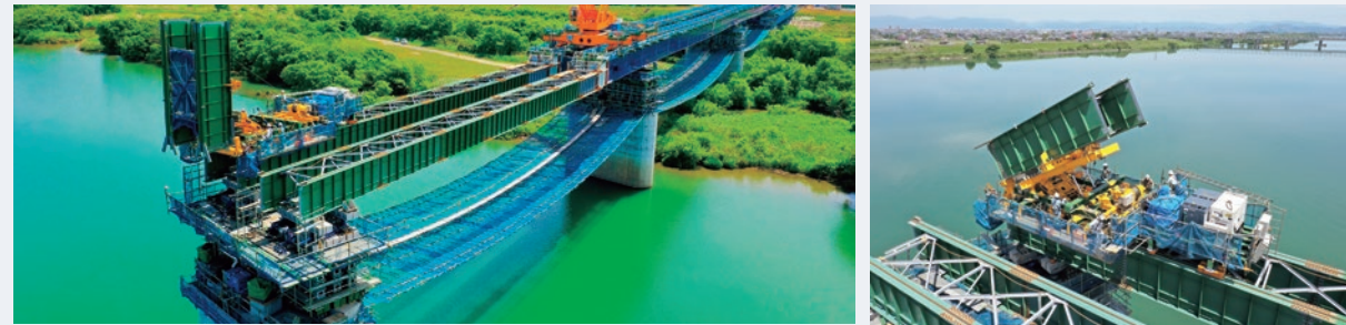
Shin-Nobi Bridge during launching gantry dismantling using the Backward-Turning Self-Propelled Launching Gantry Dismantling Device
