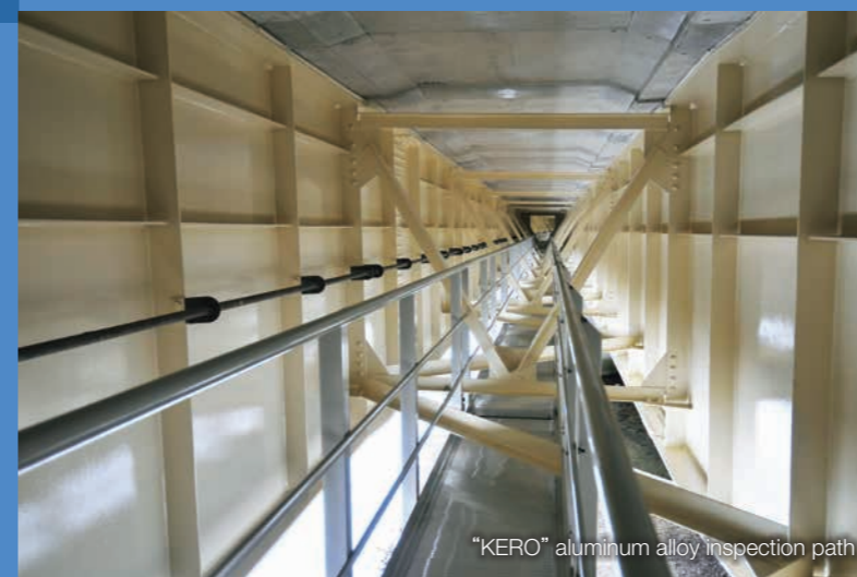
"cusa" installation on a large, long bridge (the Tsurumi-tsubasa Bridge)
